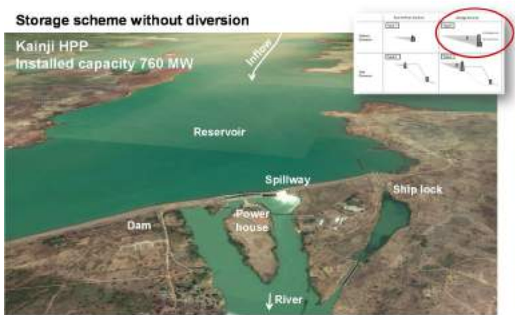
Figure 56: Hydropower plant type “Storage scheme without diversion”. Example Kainji HPP, Nigeria.
