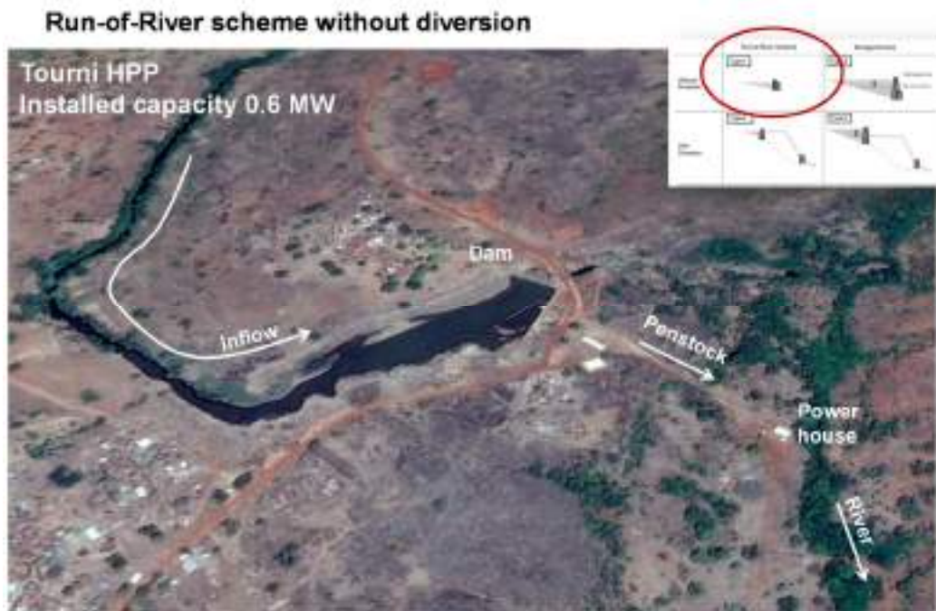
Figure 54: Hydropower plant type “Run-of-river scheme without diversion”. Example Tourni HPP in Burkina Faso.
