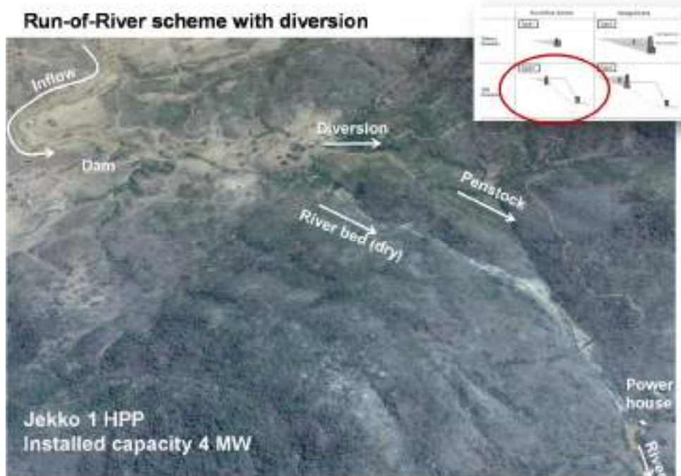
Figure 55: Hydropower plant type “Run-of-river scheme with diversion”. Example Jekko 1 HPP in Nigeria.
